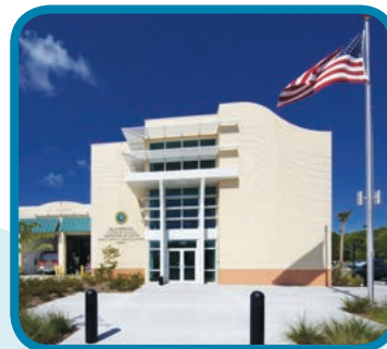
Administrative Center and Public Safety Headquarters, Islamorada, FL
