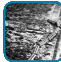
Hurricane derails train, 1935 Photo Source: Original uploader E. Brown
