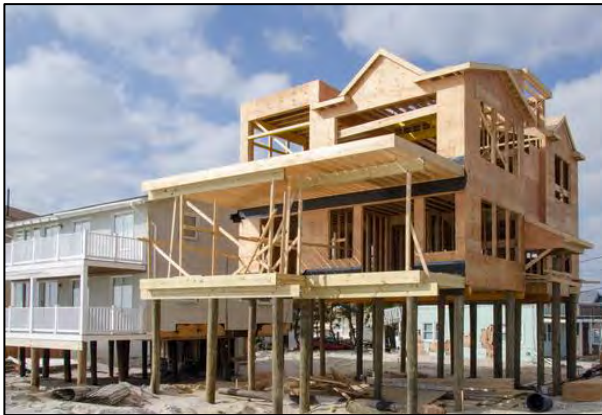
Figures 8a and 8b. Elevated house (left) and floodproofed house (right). Source: http://www.theepochtimes.com/n3/4747-hurricane-sandy-katrina-offer-similar-lessons-for-builders/
